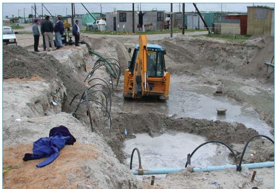
**Figure 3.** Excavating and De-watering the Site for the 1065 mm Chamber.
