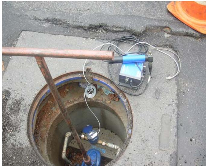
**Figure 1.4** – Specially sized meter and data logger installed on a bypass for the test
