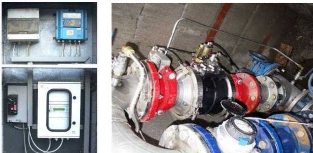
**Figure 1.2** Data loggers and a measurement point
