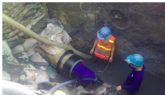
*A member of the Maynilad Leak Detection Team guides a CCTV camera into a pipe to find leak sources, while two team members spot.*
