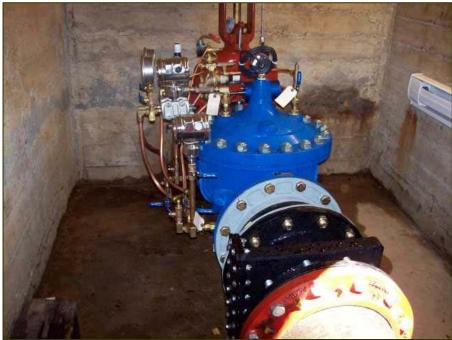
Figure 5 - Donlands & Aldwych Flow Modulating PRV Installation
