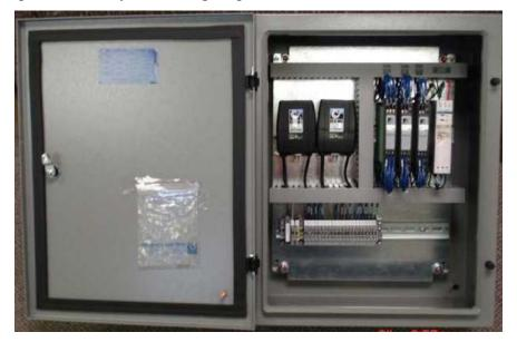
Figure 6 - PRV Control Panel & Wiring Strip
