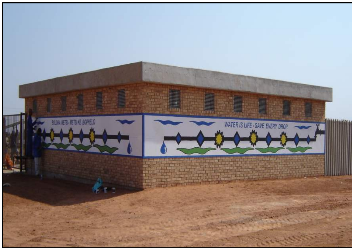
Figure 13: External view of the Sebokeng pressure management installation
