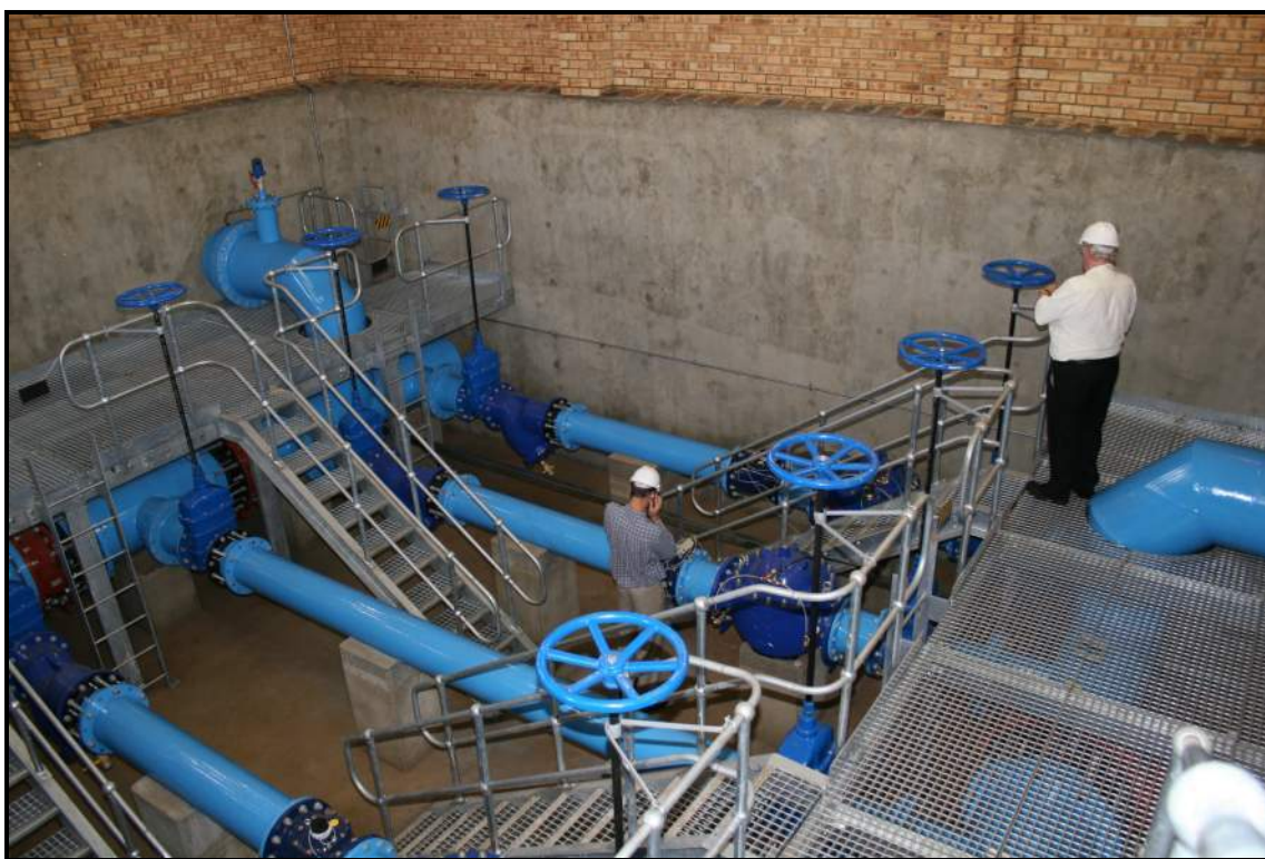
Figure 12: Sebokeng/Evaton pressure management installation
