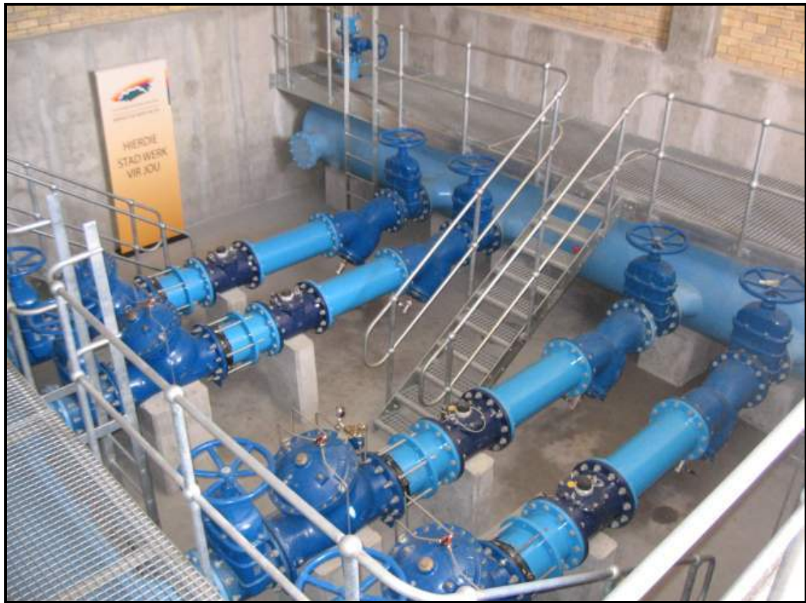
Figure 15: Mitchells Plain pressure management installation
