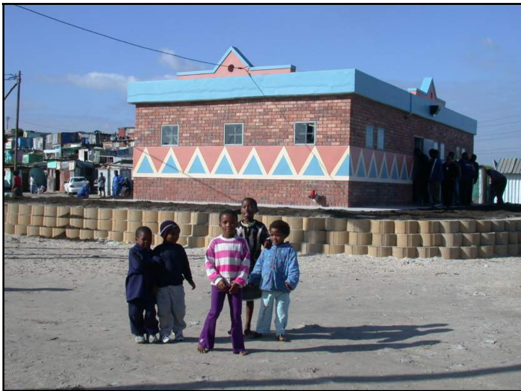
Figure 9: External view of the Khayelitsha pressure management installation
