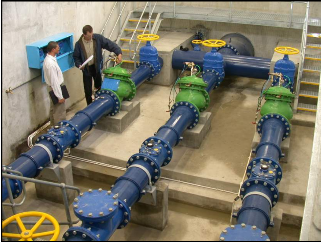
Figure 8: Khayelitsha pressure management installation
