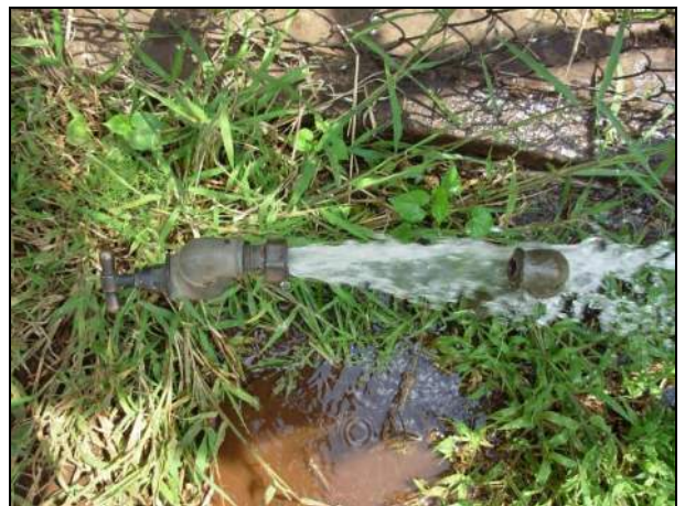
Figure 6: Photos of connections where meters had been stolen or unlawfully removed.
