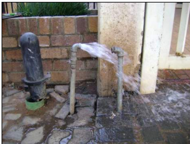
Figure 6: Photos of connections where meters had been stolen or unlawfully removed.
