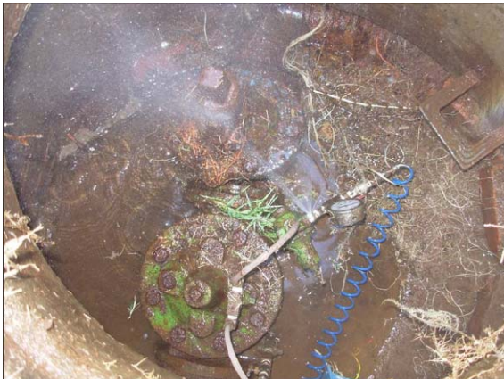
Figure 3: Pressure reducing valve installations prior to refurbishment
