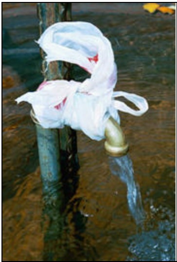
Figure 8 Leaking Tap
